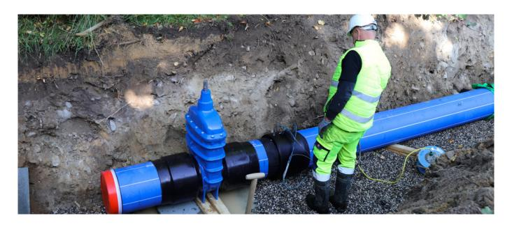
A fully welded PE pipe system offers a lot of benefits such as reduced risk of leakage, ease of installation and a high durability. We have recently launched gate valves with PE ends in four new sizes with outside pipe diameters of 450, 500, 560 and 630 mm, so with AVK gate valves with pre-mounted PE pipe ends you can now design a fully welded pipe system up to 630 mm.
