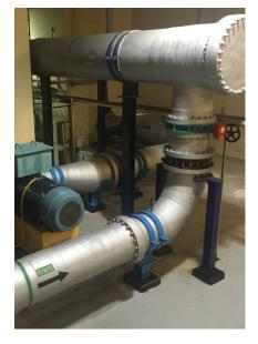
Products delivered to the project include Desponia butterfly valves from InterApp, manual and motorized from DN200 to DN600, PN16, 164 pieces in total. From AVK Anhui, series 756 motorized butterfly valves DN1600, 6 pieces.
